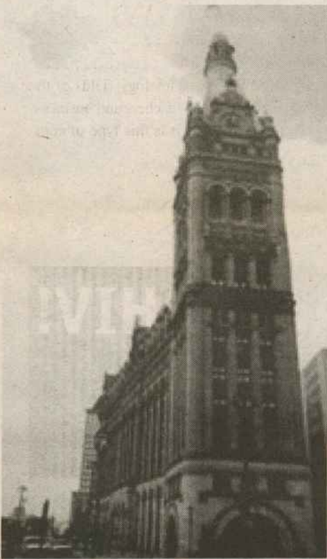
Milwaukee's City Hall
