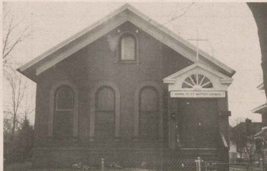
The new home of Milwaukee MCC
