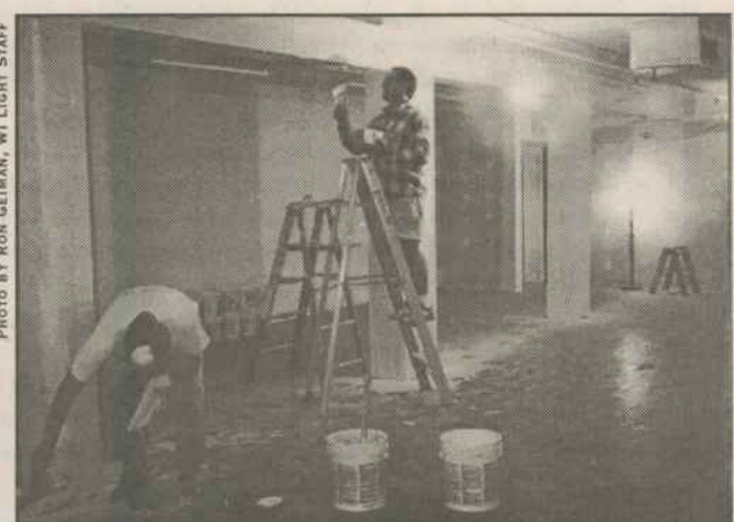
"Mudding" the joints at the new Milwaukee LGBT Community Center.
