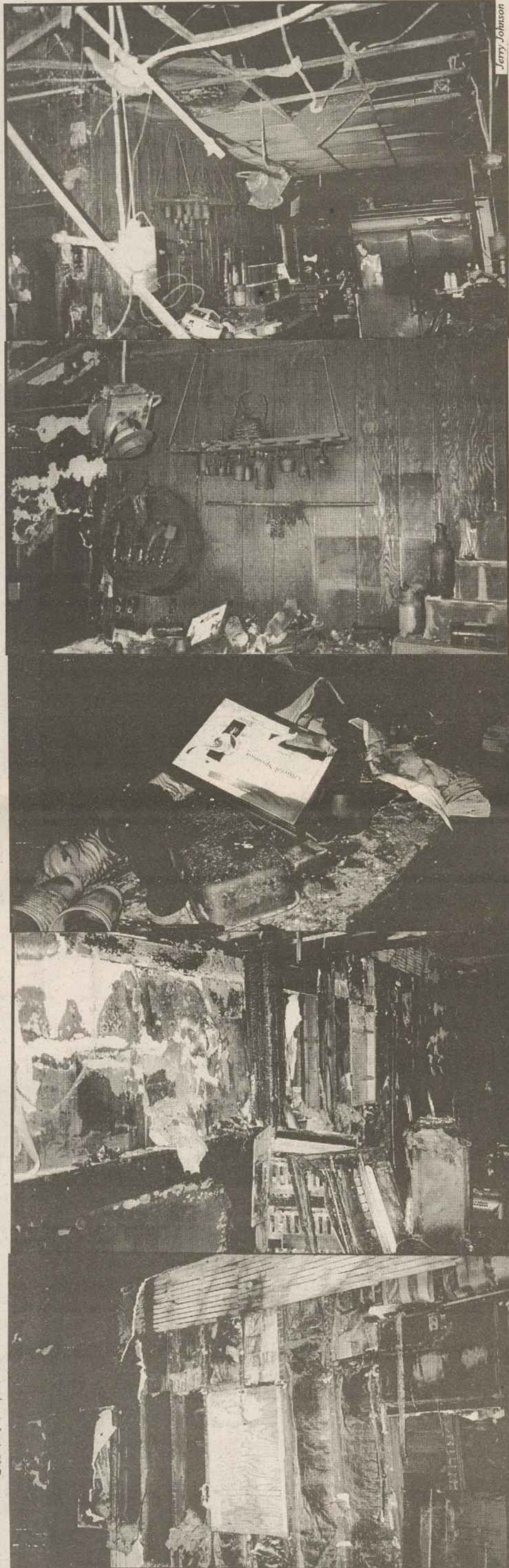
Fannies Fire Damage — Extensive fire and water damage from the arson blaze at Fannies earlier this month is shown above. Fannies owner Sharon hopes to be able to reopen the landmark Milwaukee bar.
