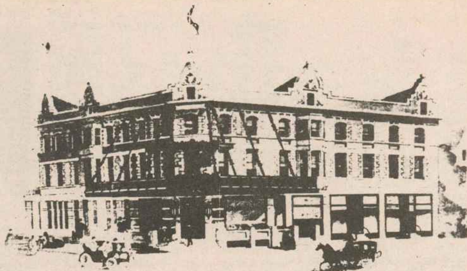
Madison's Hotel Washington as it looked at the time of its opening in 1905.
