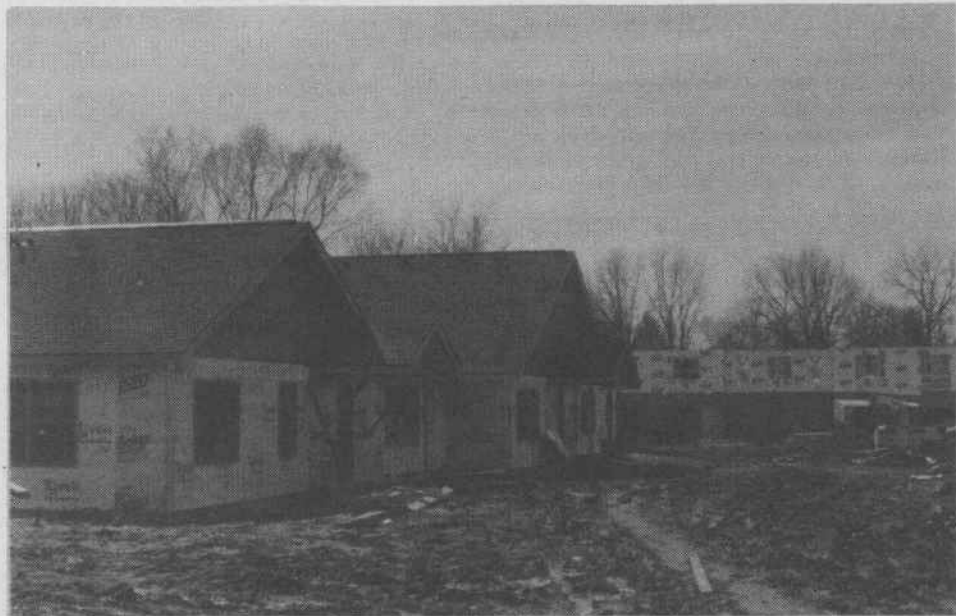
The Rodney Scheel House under construction
