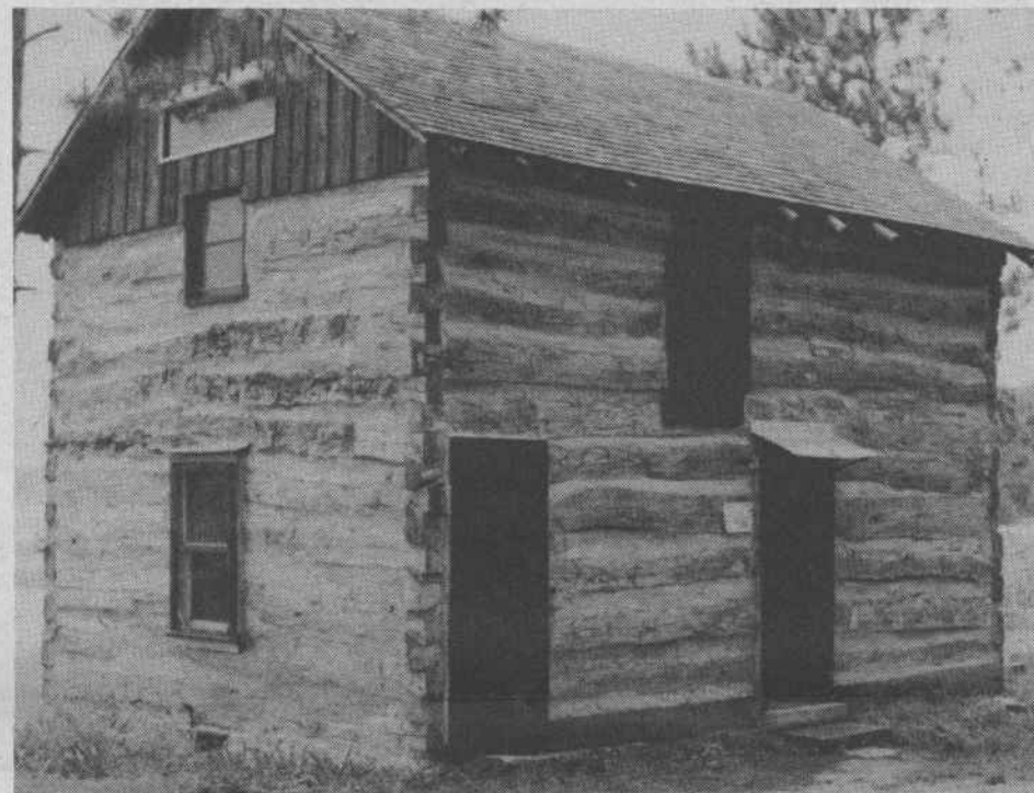
This historic two story dwelling is a part of the building collection at the Reedsburg Pioneer Log Museum. Note the dovetail construction of log joints and exposed eave beams. The roof is covered with wooden shingles and the top, front window is shuttered. This house once served as the Oetzman residence.
