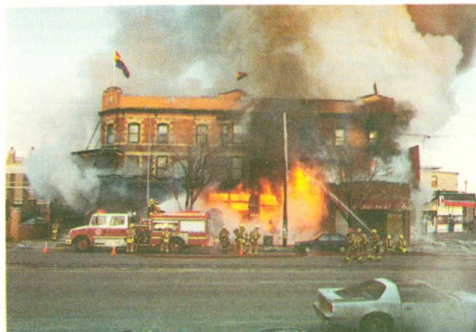
Landmark Levelled—Fire quickly raged out of control and engulfed the entire Hotel Washington on February 18 th .
