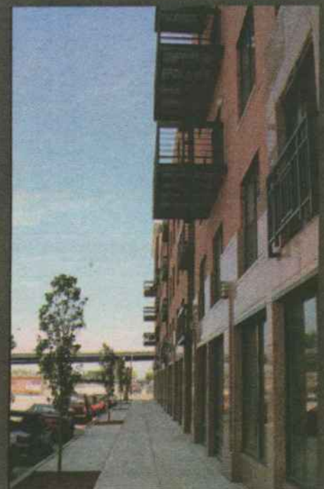
Jefferson Block apartments 144 N. Jefferson Street
