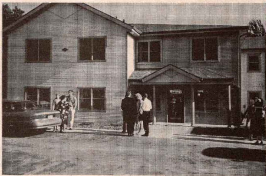
The Rodney Scheel House for PWA's in Madison held an Open House on July 18. Photos by John Cain.
