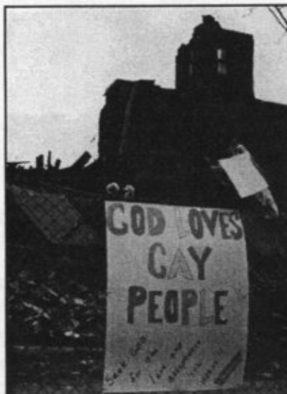
A huge rainbow flag was draped over the Hotel's only standing wall, and people left memorabilia and messages on the fence surrounding the site.
